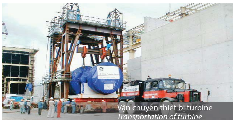
Lắp đặt turbine Erection of turbine
